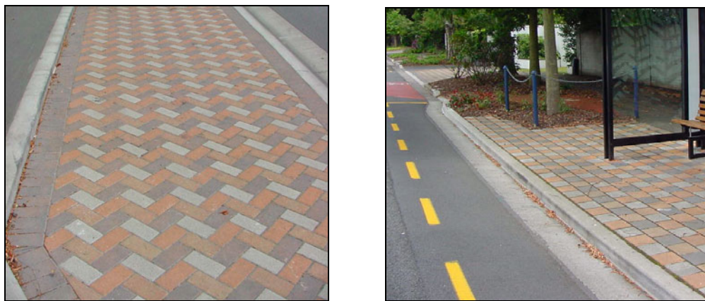
Cobblestone paving laid to herringbone and staggered patterns
