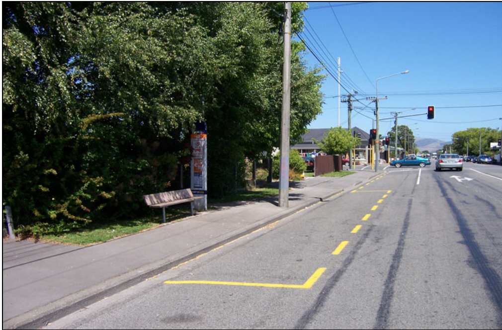
Typical kerb side bus stop in Christchurch
