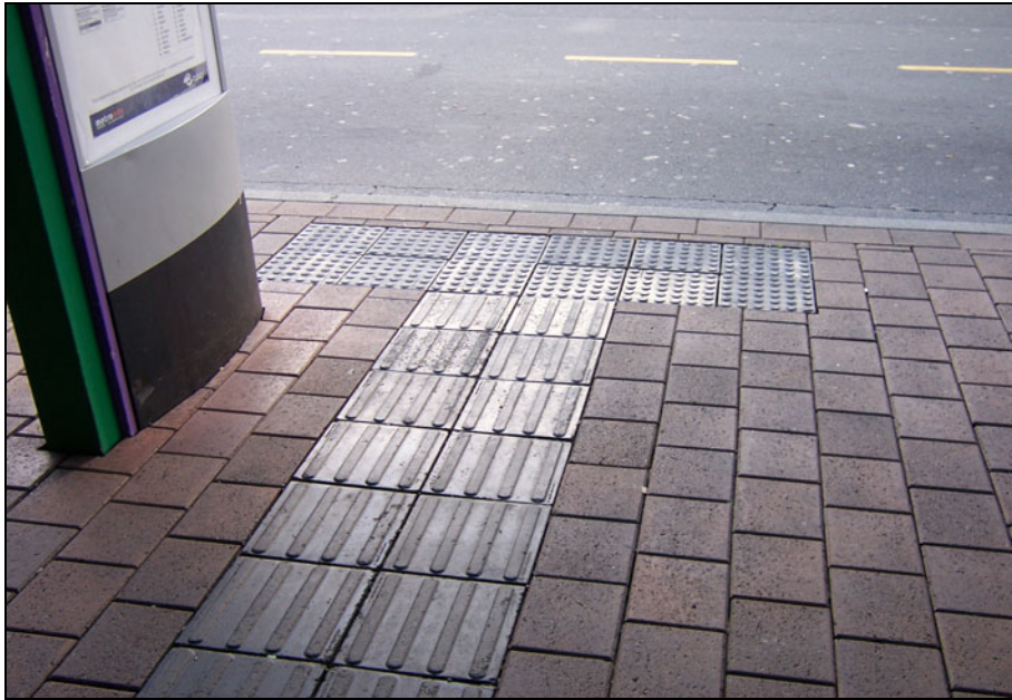
Directional and warning indicators at a bus stop, Colombo St
