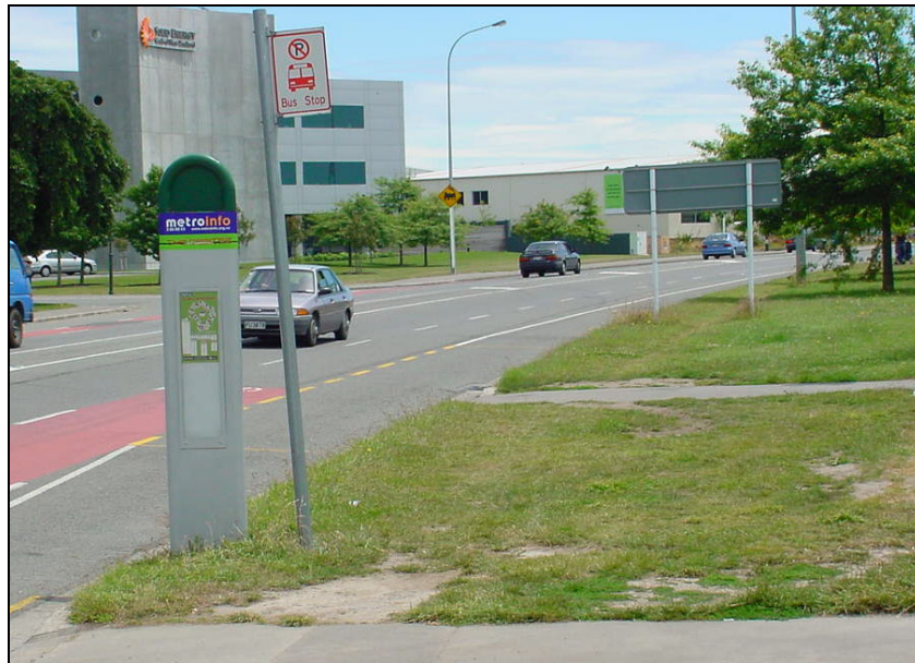
Unsealed passenger areas make access difficult for elderly and mobility impaired passengers
